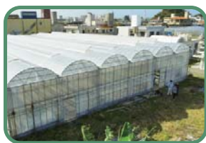
結構力霸型溫室 Robust Structure Greenhouse
